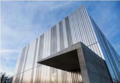
Building for a data centre in Basel, Switzerland
