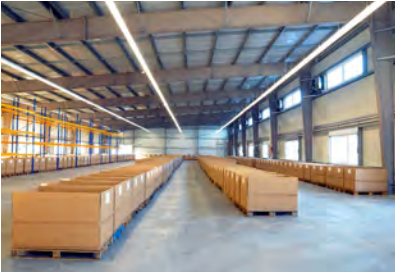
Logistics facility in Fürstenwalde, Germany
