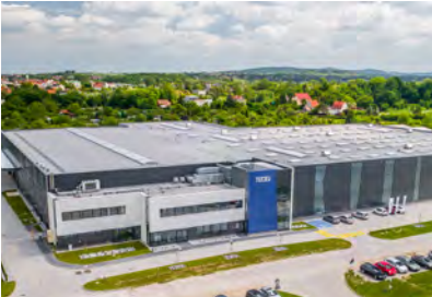
Production and warehouse facility in Strzelin, Poland
